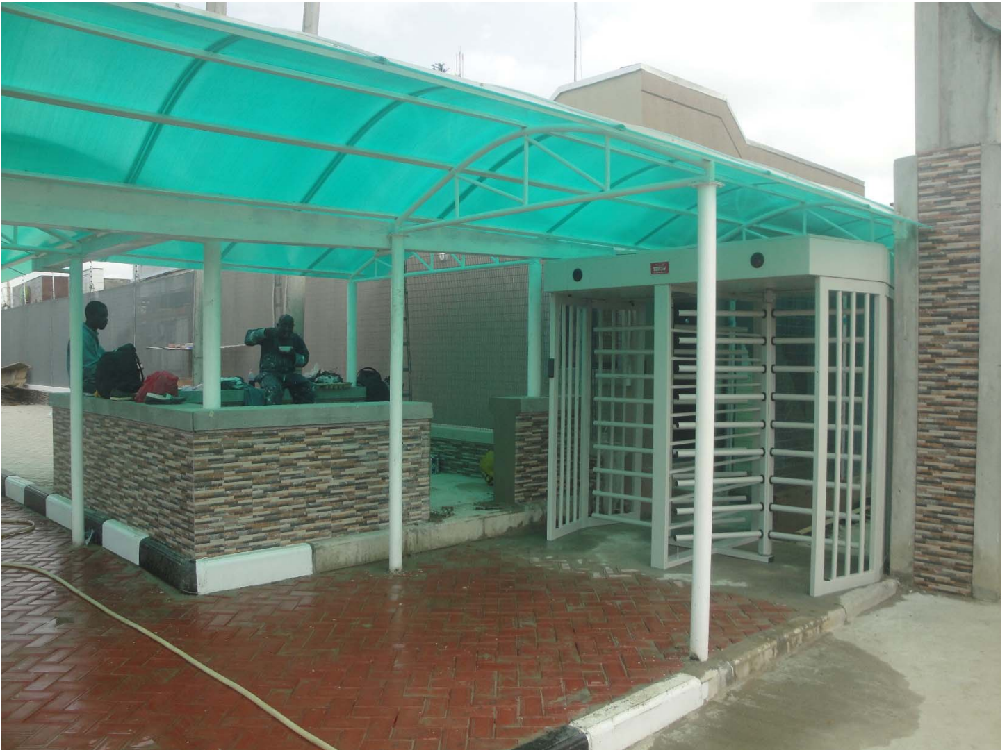
Covered office entrance in Nigeria, Africa: (1) TTF400 Series
