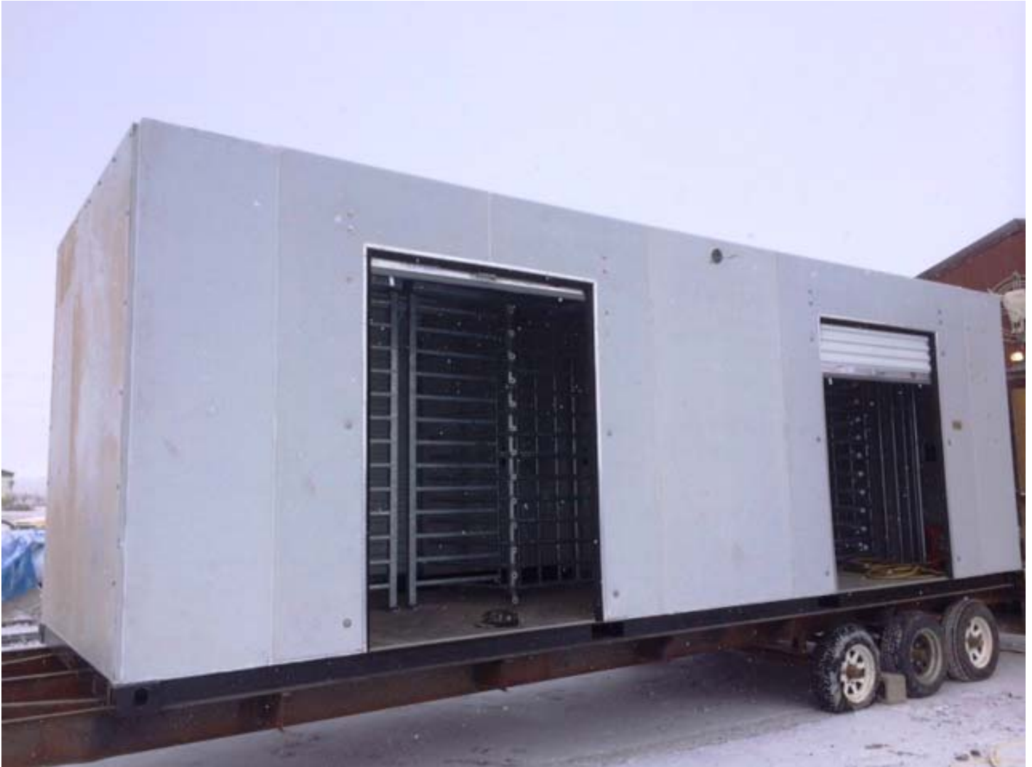
Portable building for temporary entrance on a construction site.
