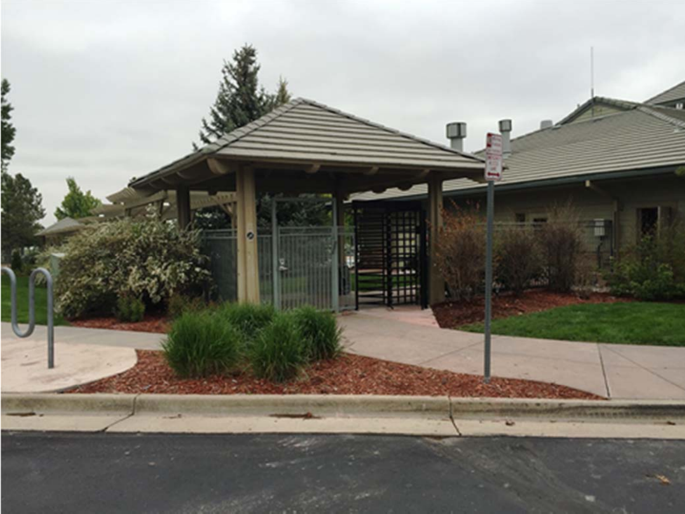
Installation at community center in Colorado: HS430-PC Black with ADA Gate
